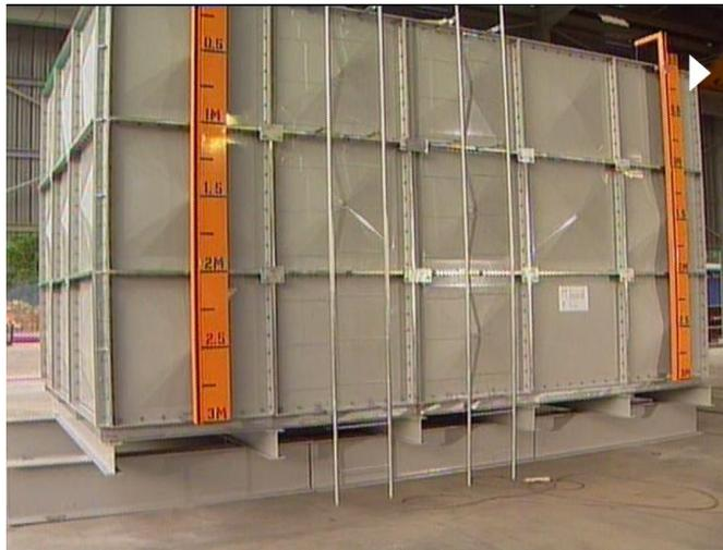
GRP panels tanks are installed and fitted with complete accessories to include internal PVC ladder, external galvanized steel ladder, level indicator, air vents, access manhole and supported either by the stainless steel tie rod internally or galvanized box sections externally.
