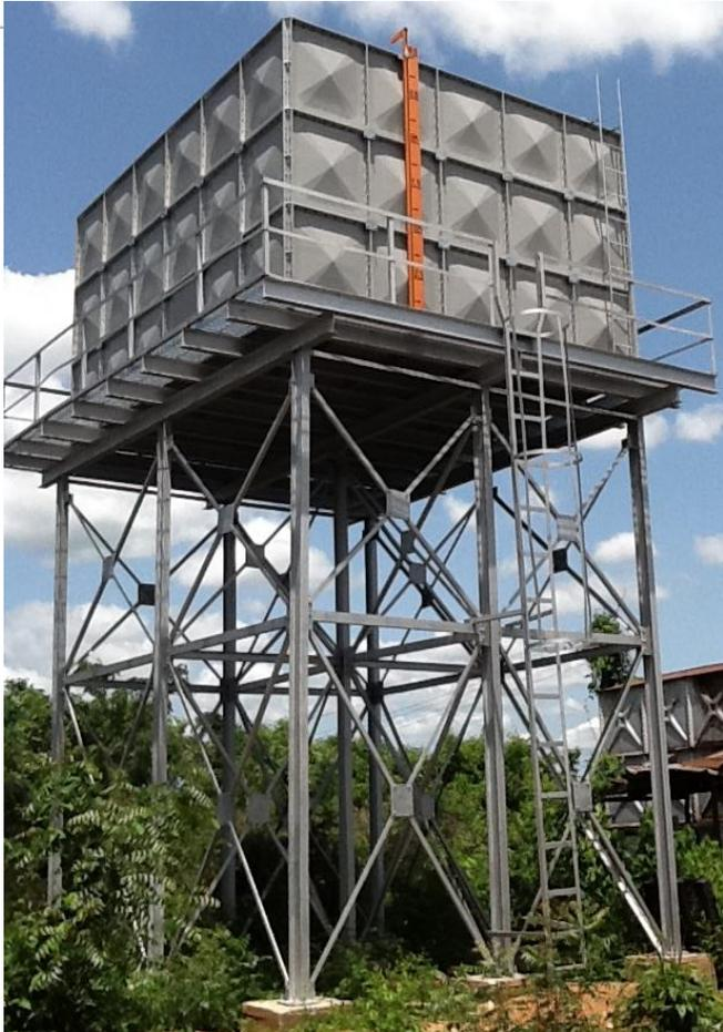
The GRP tanks are manufactured from non-corrosive materials and as a consequence require little or no specific maintenance other than routine checkup which can be done once a year.
