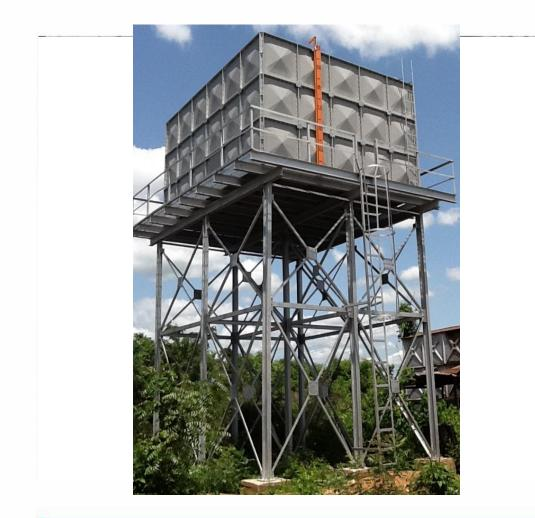
The GRP tanks are manufactured from non-corrosive materials and as a consequence require little or no specific maintenance other than routine checkup which can be done once a year.
